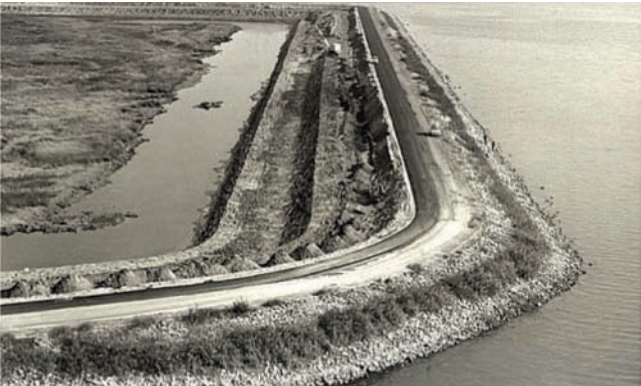
Defense embankments to protect against erosion in the Sacca degli Scardovari.
