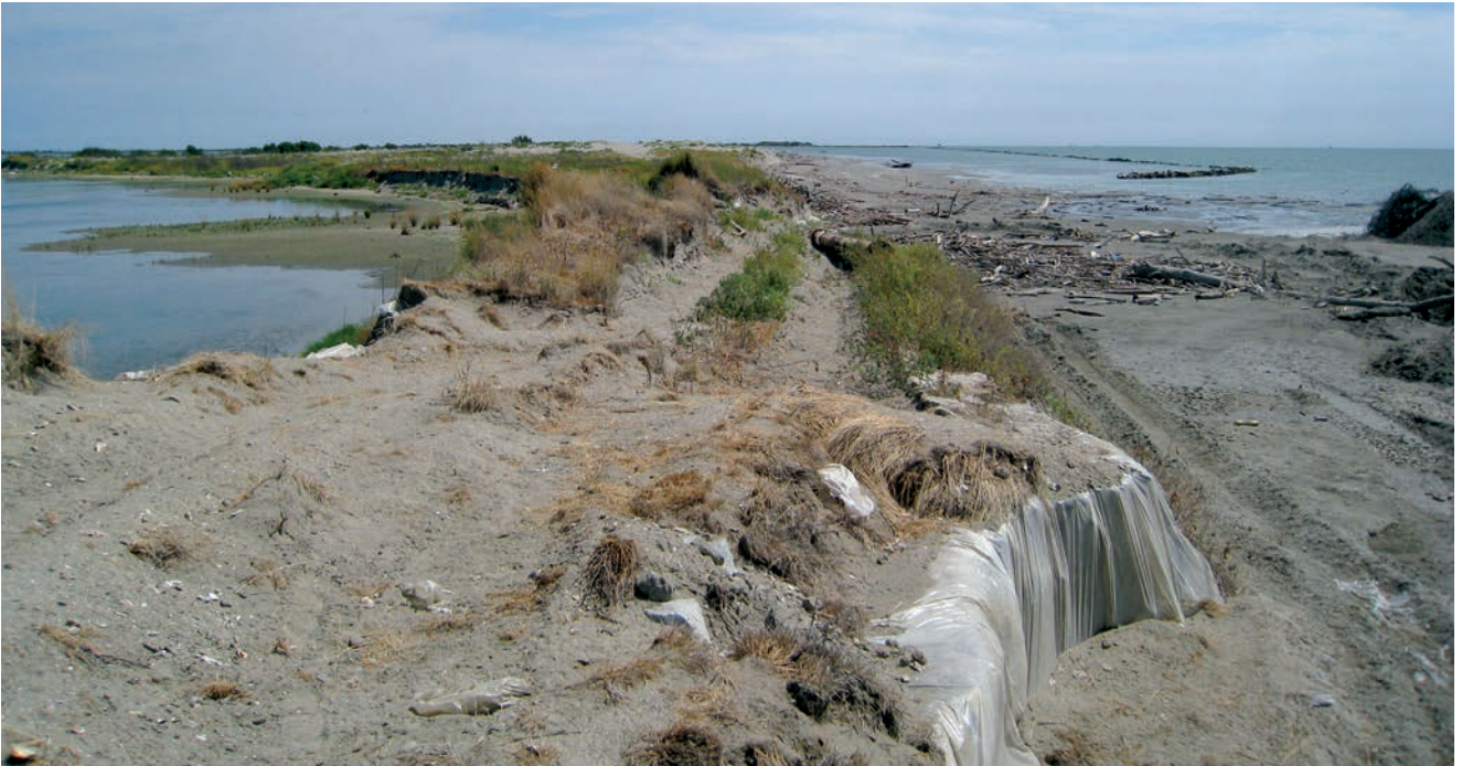
Figure 4: in the foreground one can clearly see the small earthy diaphragm, with its plastic film reinforcement introduced during construction separating the beach from the lagoon, covered with sparse ruderal vegetation. On the lagoon side (left), the presence of intertidal transition surfaces can be noted. This photo dates back to 2009; the sea facing artificial beach is now much larger as a result of recent ebb flow (photo: Bonometto 2009).
